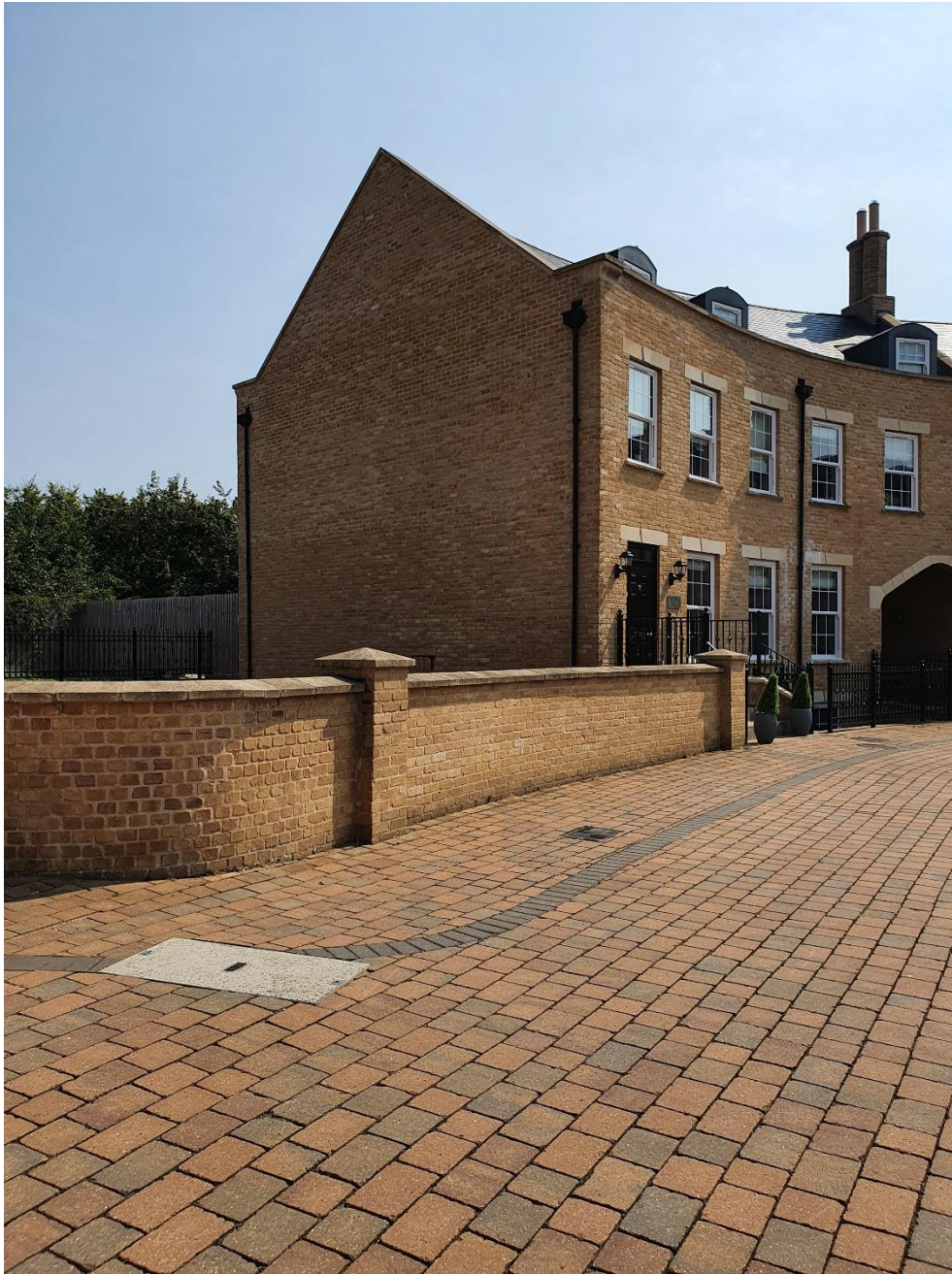
The end gable of No. 19
